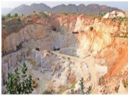
A quarry in operation in the core area of the Sariska tiger reserve. Jay Mazoomdaar
