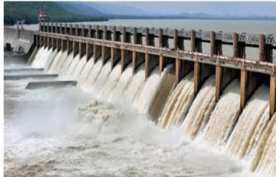
Emergency action: The remaining 32 crest gates of the dam were opened to reduce the pressure on the broken gate. SRIDHAR KAVALI
